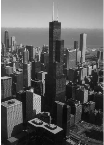
At 1,454 feet, the Sears tower was the tallest building in the world until February 1996.
