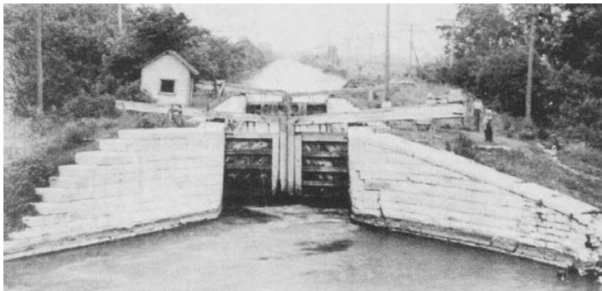
Locks on the Illinois and Michigan Canal at Marseilles.
